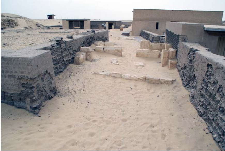
FIGURE 57 The anonymous chapel 084/USC built in the passageway between the tombs of Ptahemwia (025/USC) and an anonymous official (082/USC) PHOTOGRAPH BY THE AUTHOR, 2017
